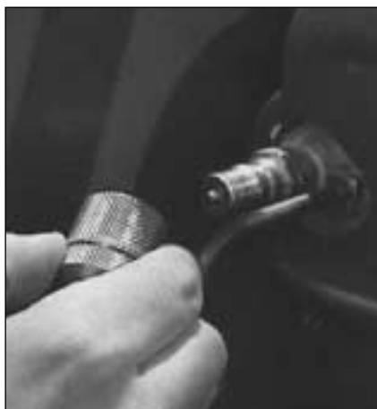
Modular switch / CB filler point
